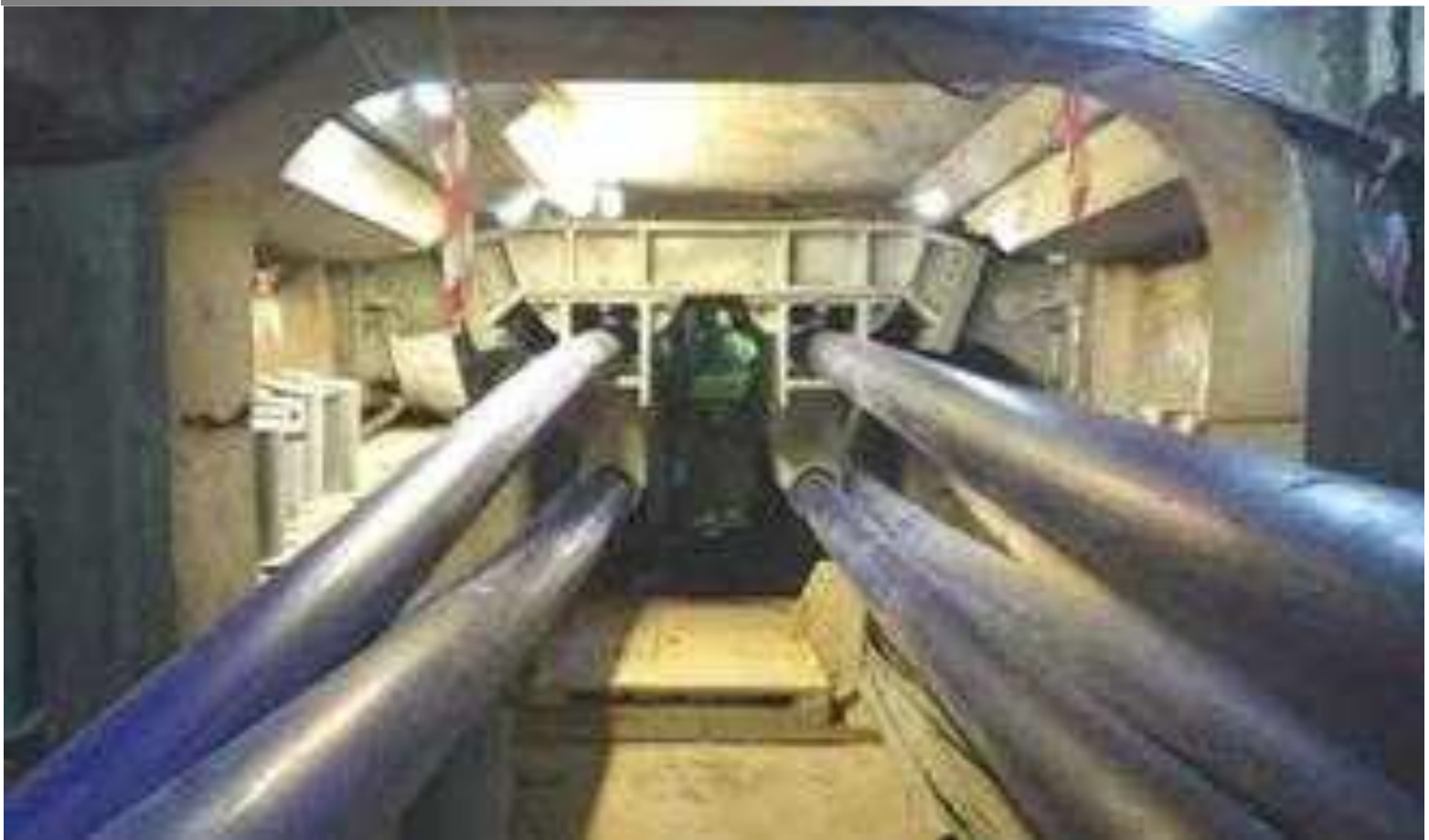
Access constraints while fitting the new tensioning tendons (HSE, 2018)
